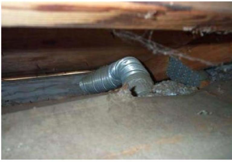
This bathroom exhaust fan does not exhaust to outdoors – just to the soffit.
