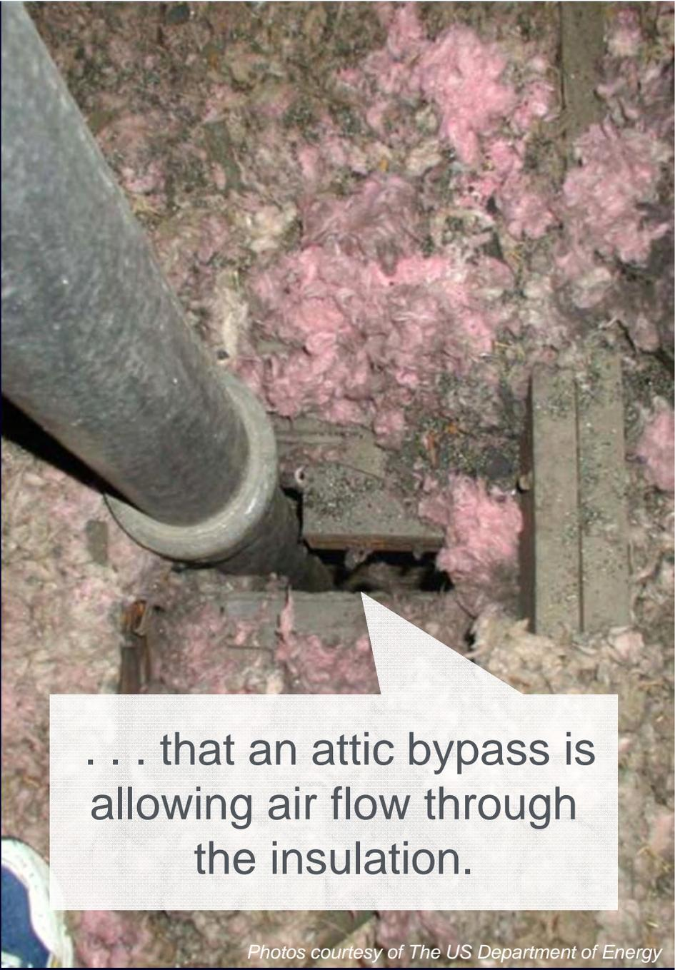
. . . that an attic bypass is allowing air flow through the insulation.
