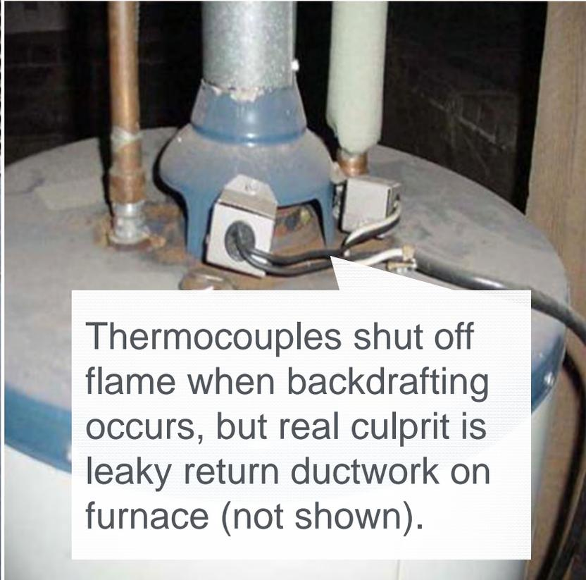
Thermocouples shut off flame when backdrafting occurs, but real culprit is leaky return ductwork on furnace (not shown).
