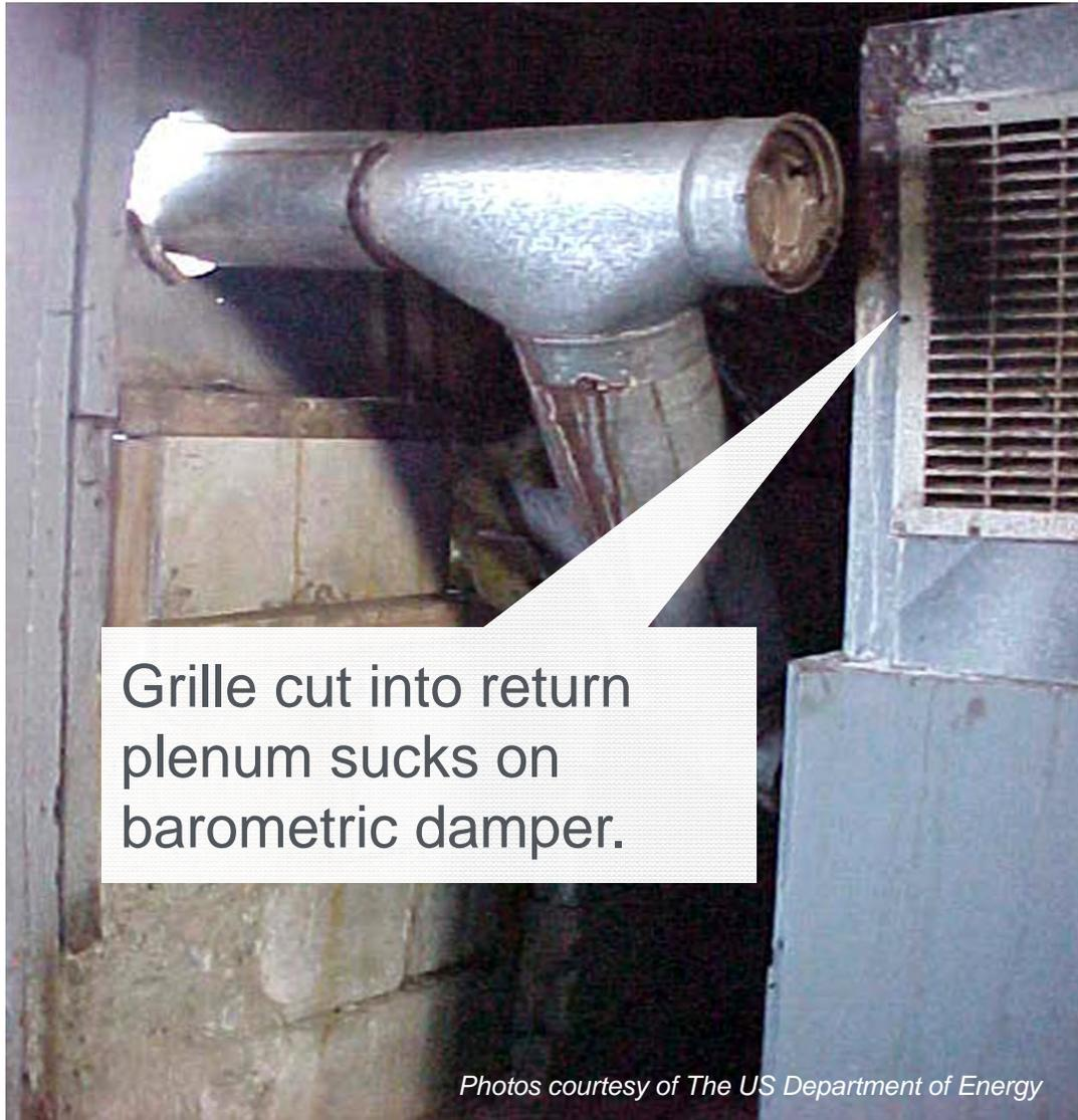
Grille cut into return plenum sucks on barometric damper.
