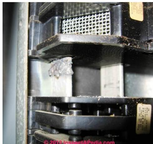
**Fig. 9. Burned Zinsco™ Circuit Breaker.**
