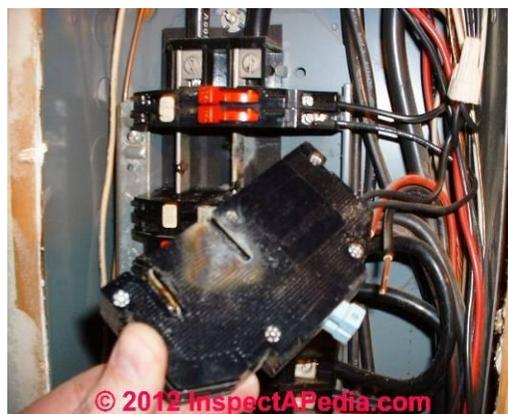
**Fig. 8. Zinsco™ Double-Pole Thin Style Breaker, Light Green Toggles, with Burn and Arcing Flash Marks.**
