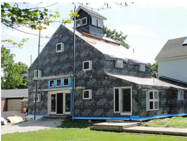
**Photograph 8: Fully Adhered Membrane**—Ultra high levels of airtightness with ultra high levels of cost. Not the easiest stuff to install either. I should know, this is my place.
