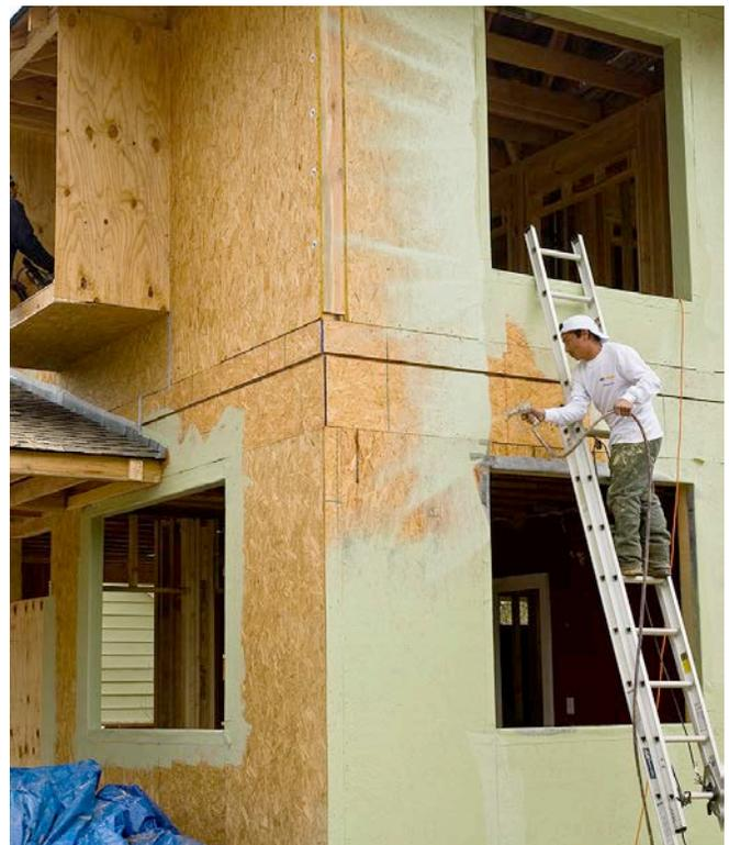
**Photograph 9: Fluid Applied Air Barrier**—The coatings needed to be able to span joints and they needed to be vapor permeable. And their most important function, rainwater control could not be compromised.
