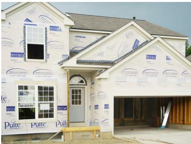
**Photograph 5: Air Infiltration Barrier**—Classic housewrap rainwater control layer and air control layer. Note the beautiful job of flashing integration with the housewrap. The outside is the right place for air control.
