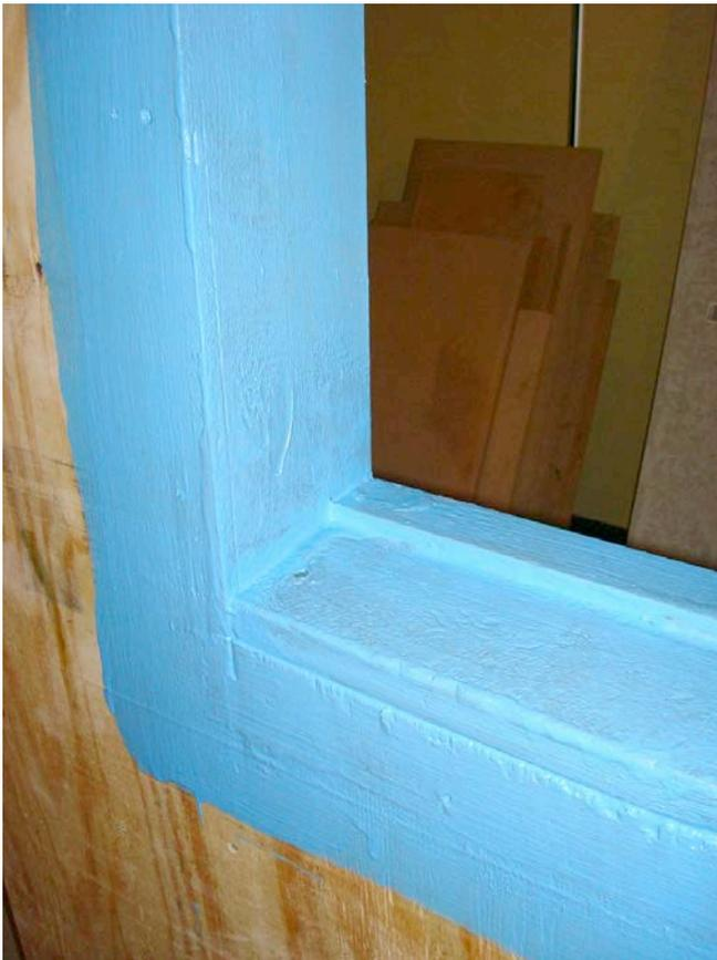
**Photograph 11: Window Opening—** Origami is not a necessary skill with fluid applied flashing systems.
