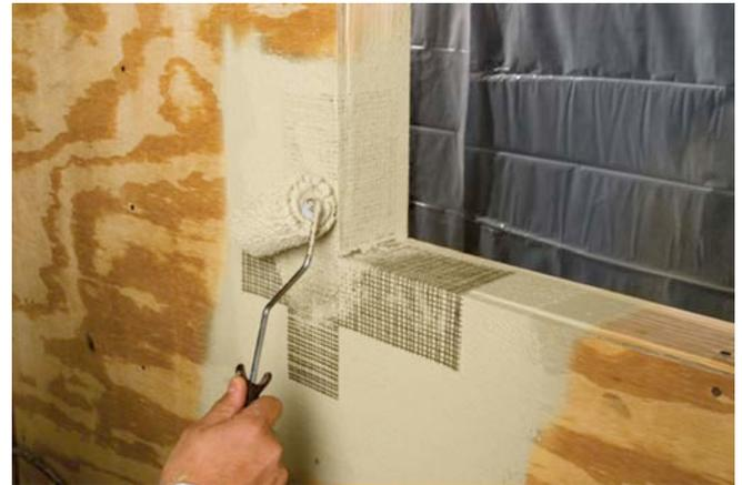
**Photograph 12: Another Window Opening—** Some systems require fabric reinforcement at critical interfaces.
