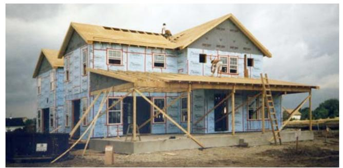
**Photograph 14: Insulating Sheathing Water and Air Control Layer—** The insulating sheathing provides three functions in this approach – water control, air control and thermal control.
