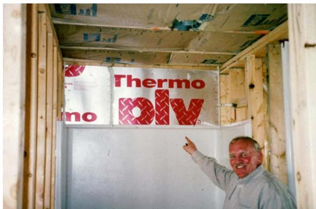
**Photograph 4: One-Piece Tub Shower Enclosures**—A really, really big hole on an exterior wall sealed by a very happy builder. Note the sealant around the perimeter of the rigid draft-stopping sealing the draft-stopping to the framing.
