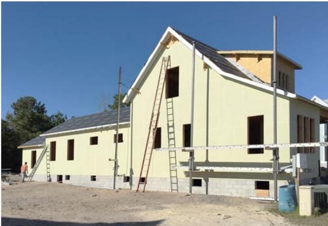
**Photograph 10: Water Control/Air Control Continuity—** The fluid applied coating must connect to the air control layer of the roof assembly and to the air control layer of the foundation assembly.
