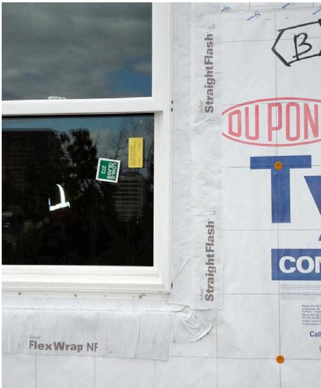
**Photograph 6: Robust Rainwater Control**—Numerous elegant and clever accessories were introduced to deal with rainwater control particularly at window-to-wall interfaces. This is a formable and flexible membrane “pan flashing” system.
