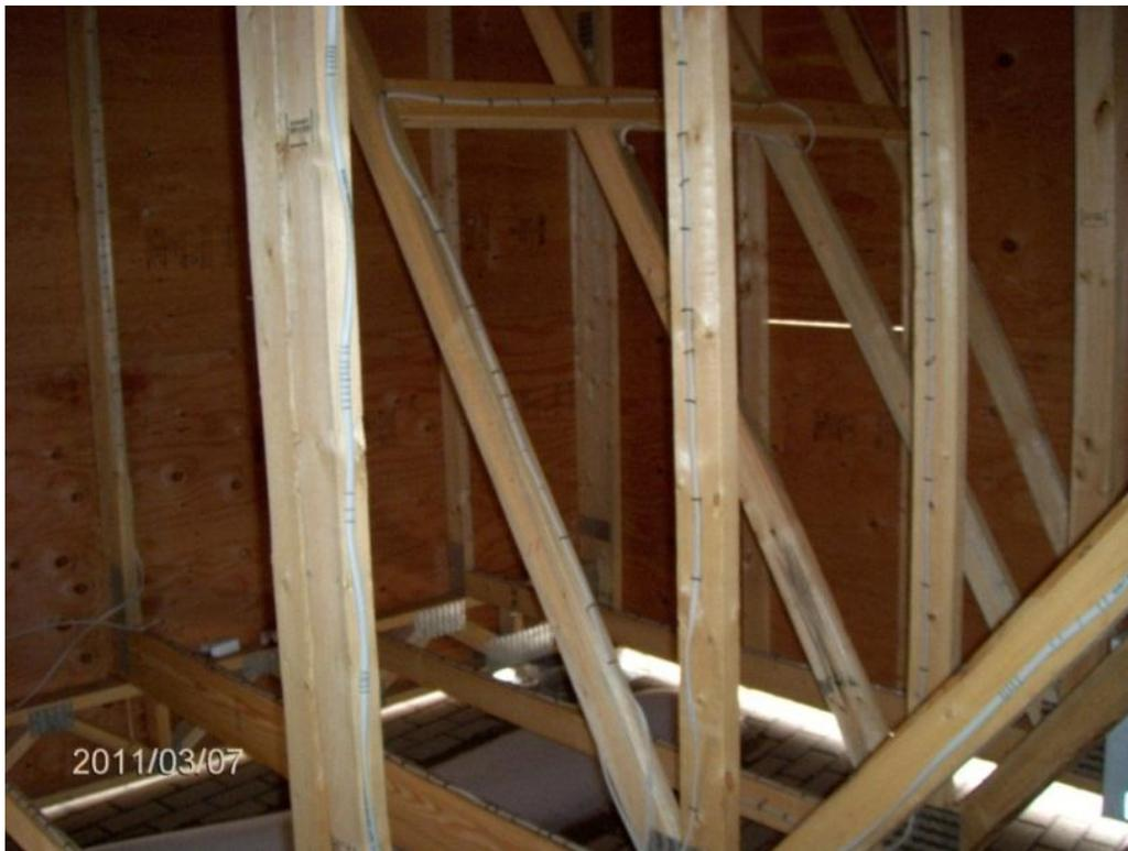
Figure 19 - NM cables installed on wood studs
