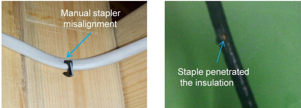
Figure 20 - NM cable damaged by misaligned staple
